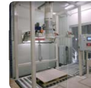
➤ Dosing and weighing: automation and ergonomics of filling station
