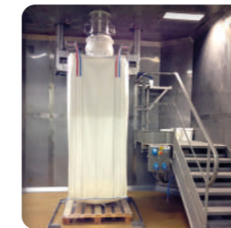
▶ Suspended structure facilitates floor cleaning
