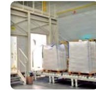
Conveyor and automation
