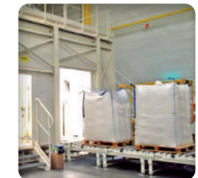
➤ Conveyor and automation
