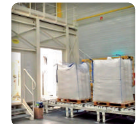
Conveyor and automation
