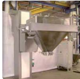
Mixer in pharmaceutical plant
