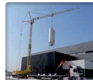
Crane and Installation on your site
