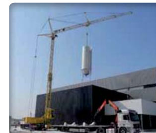
Crane and Installation on your site
