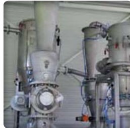
Under cyclone, resin transfer
