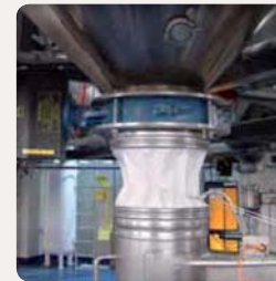
Fitting below butterfly valve with vacuum resistance
