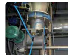
3 Dosing system for incorporation of lime
