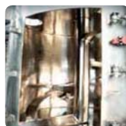
Polishing of welded components for hygienic finish
