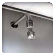
Clean In Place (CIP)
