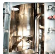
Polishing of welded components for hygienic finish
