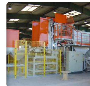
▶ Plastic injection plant
