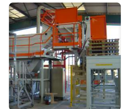
▶ Feeding of the plant by extrusion
