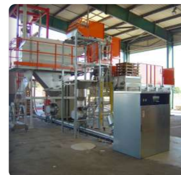
▶ Sack opening line at a polyethylene manufacturer
