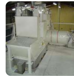
Hopper to add additives: pre-weighed and half sacks
