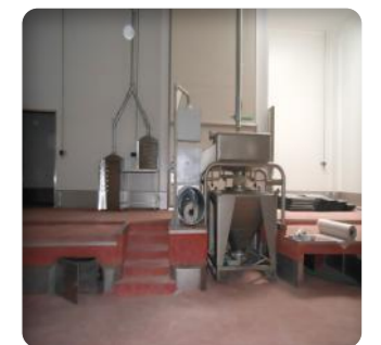
Room for pre-weighing
